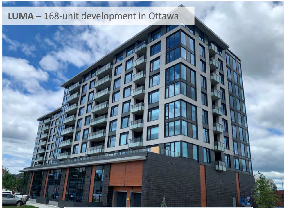
Progress shots as of June 2022
